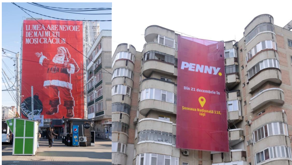
Fig. 11 Buildings covered in huge ads
