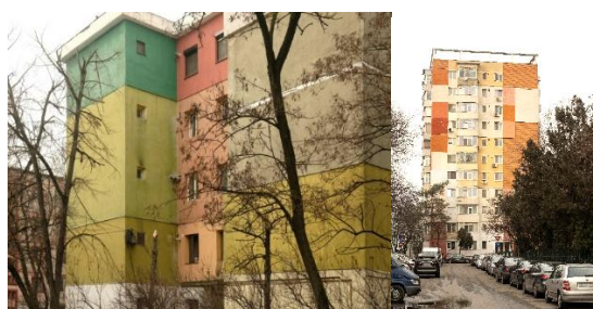
Fig. 2 Aesthetic dissonances caused by the fragmented renovation of residential buildings
