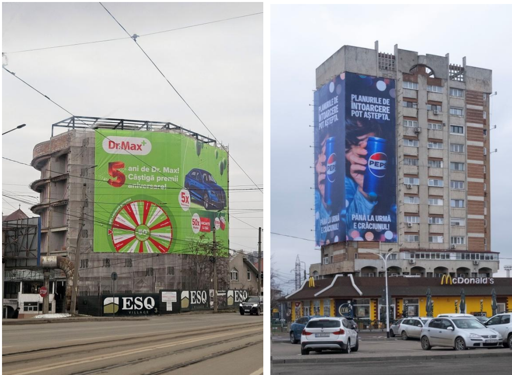
Fig. 10 Buildings covered in huge ads
