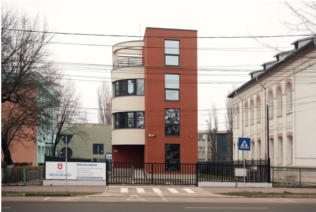
Fig. 3 Eclectic urban area caused by architectural interventions
